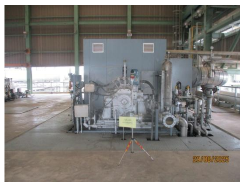
Propylene Compressor (R-650)
